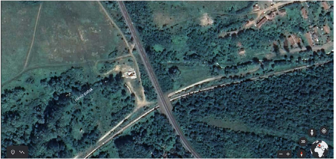
Figure 27 Road No. 2 crossing of the Hévíz-stream with an inappropriately sized culvert on Google Earth
