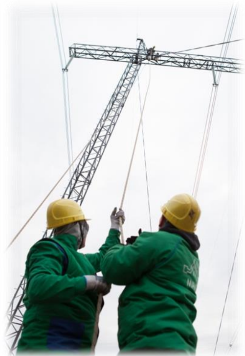
Live line nest installation
